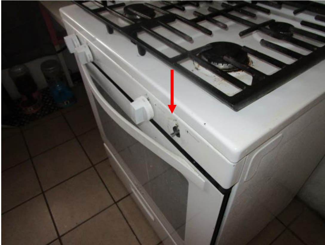
Missing range control knob needs to be serviced
